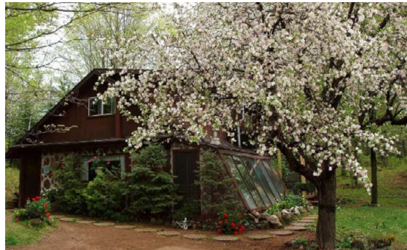
Above: The Flatau's cordwood home in lovely Wisconsin. The first floor is cordwood construction while the second is what Richard describes as "space gaining, room-in-the-attic truss."
