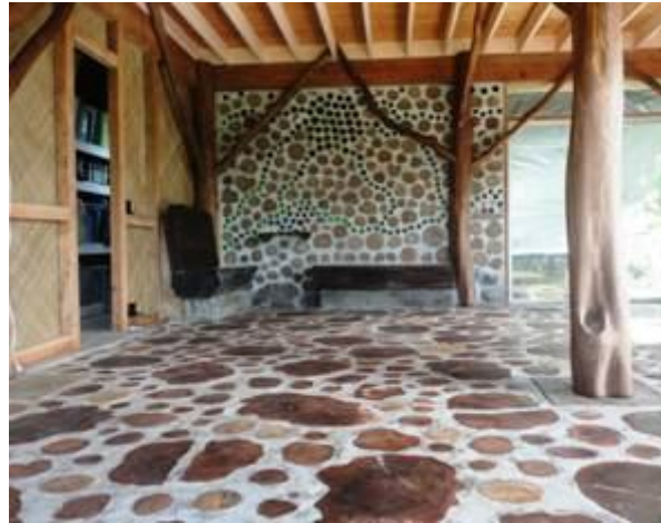
A cordwood floor – and wall - at La'akea Community near Pahoia Hawaii, mostly Ohia and Captain Cook Pine. Tracy Matfin photo.
