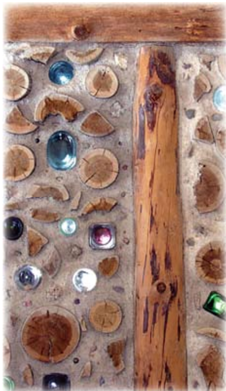
Recycled bottles were incorporated into the wall at various places to create a stained glass appearance.
